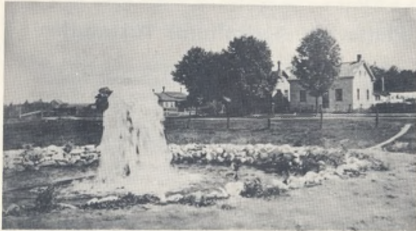
FLOWING WELL, CAPACITY 2500000 GALLS. PER DAY
